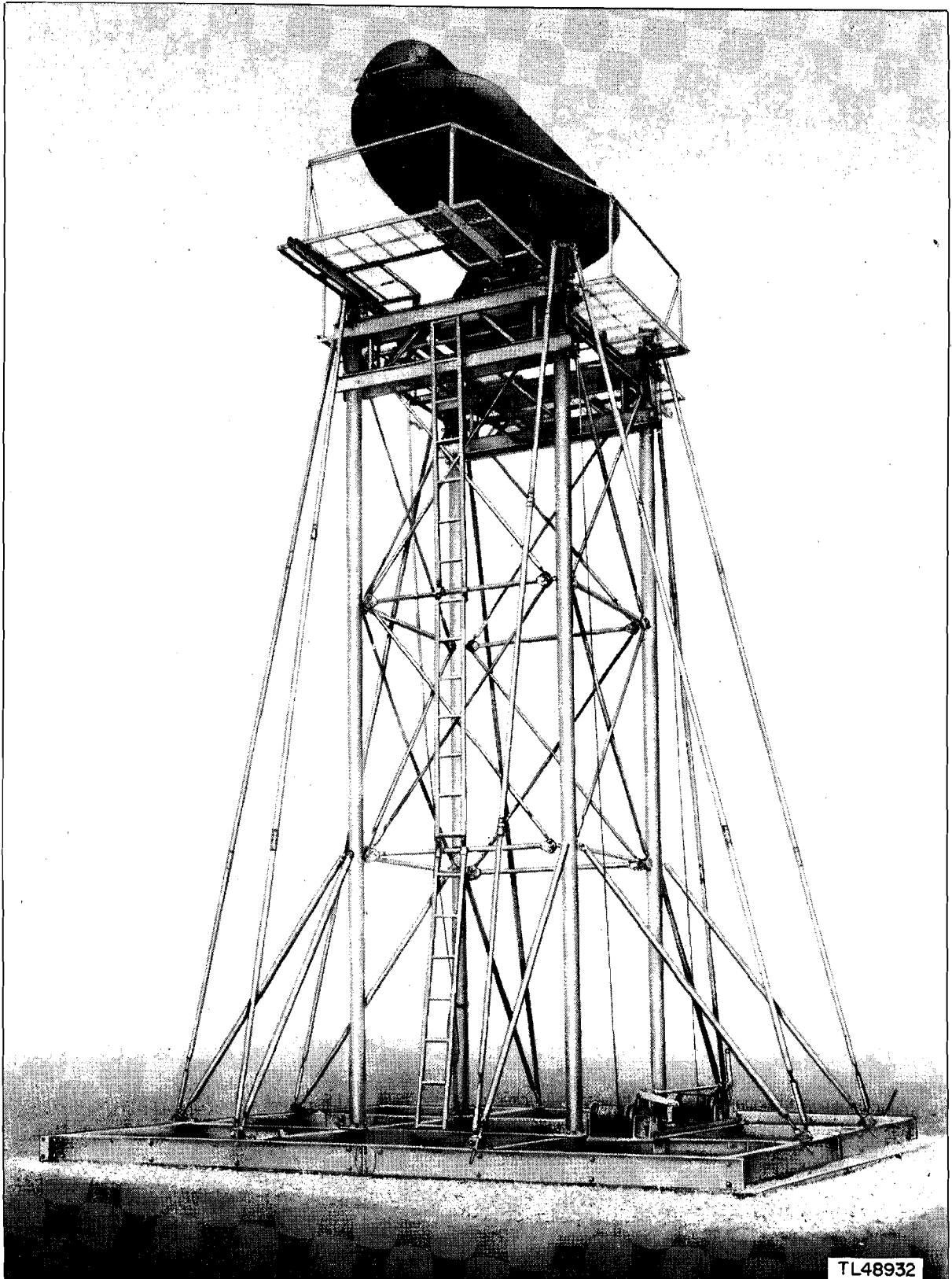
Figure 2-34. Tower completely erected.
